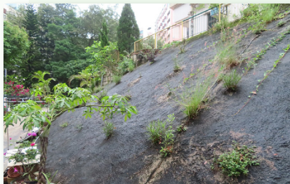
▲ Before slope improvement works
