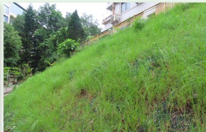
▲ After slope improvement works
